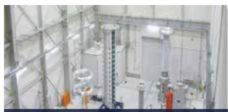
High Voltage Hall
