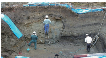
Field survey of faults by CRIEPI experts
