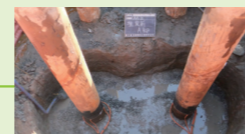
Observation of behavior of steel pipe pile foundation
