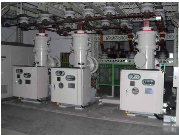
Photo 1 Making switches (three phases)
