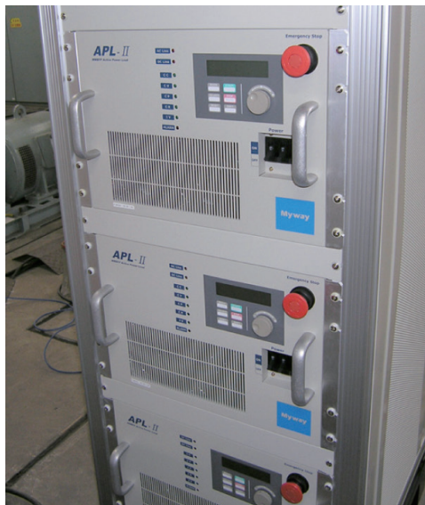
Photo 1 DC power supply emulating photovoltaic cells
